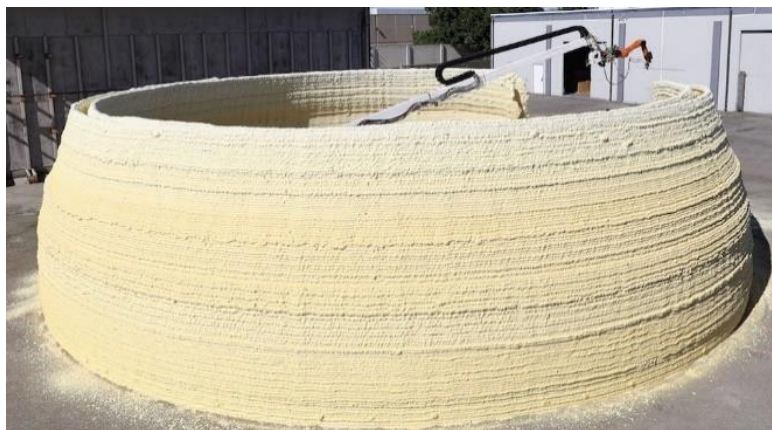
Figure 2 - Polyurethane insulation frame of a building
