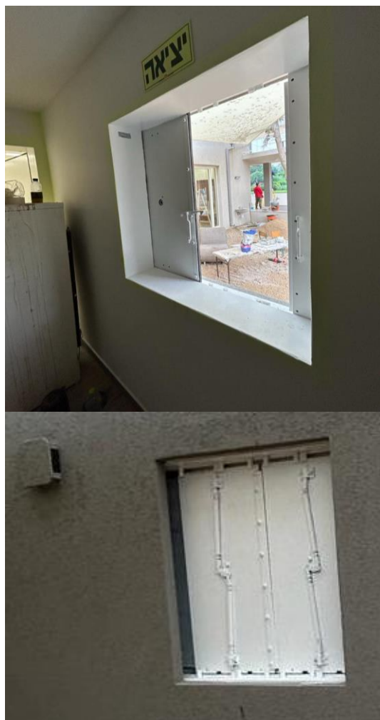
Figure 4 – Example of the implementation of a protected window opening.
