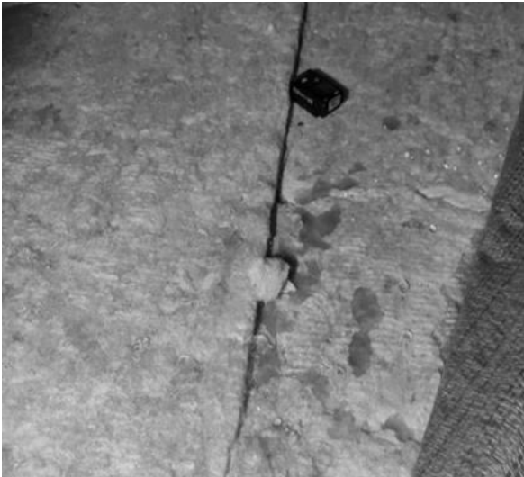
Figure 6- Location of logger №1 on mineral wool attic insulation
