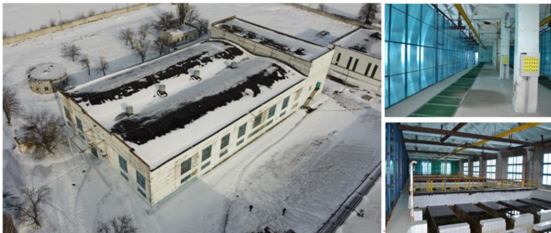
Figure 2 – General view of the building
