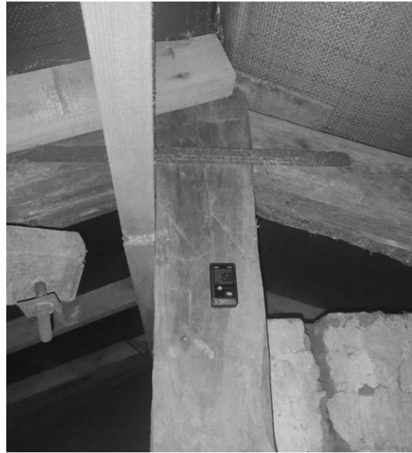
Figure 7 - Location of logger №2 under the ridge board of the roof system
