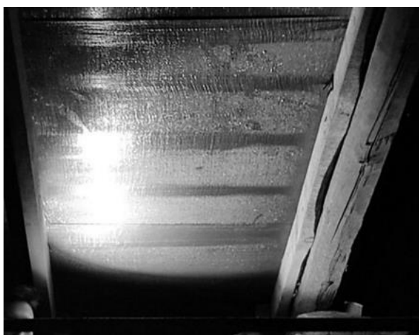
Figure 2 - A waterproofing film membrane is installed above the rafters
