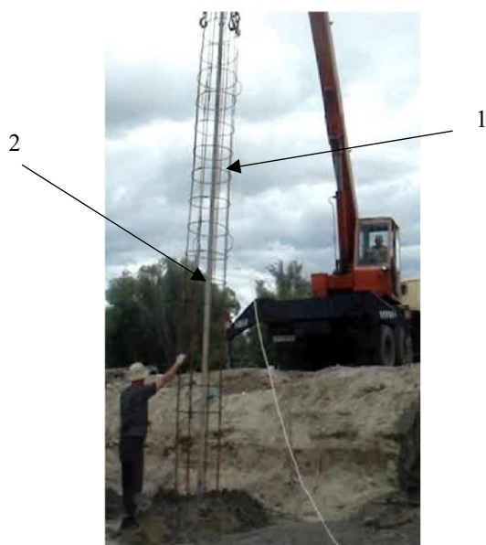
Fig. 2. – Reinforcement Cage Immersion Scheme: 1 – reinforcement cage; 2 – deep vibrator.
