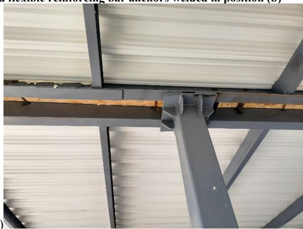
Figure 7 – General view of the support arrangement – the secondary steel beams – of the continuous cast-in-place reinforced concrete floor slab from below
